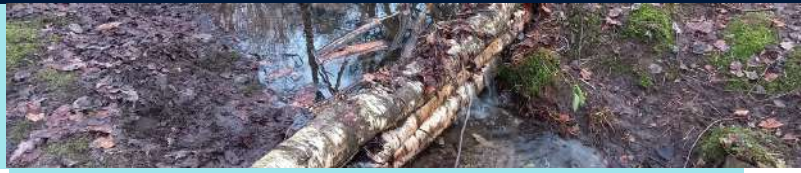
Credit: , Trent Rivers Trust, picturing leaky barriers in the Moat brook area in high flow
