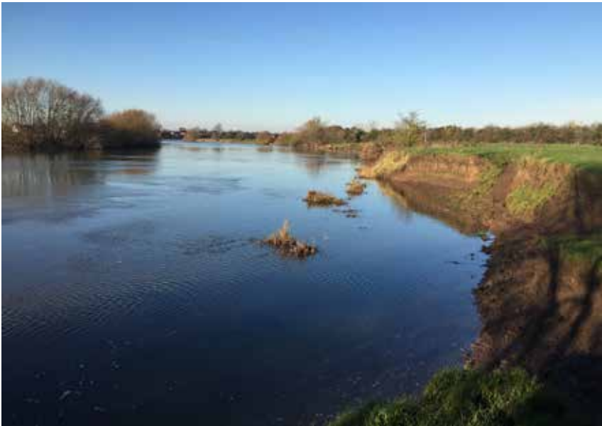
Example of lack of vegetation along river bank leading to gradual erosion of the bank
